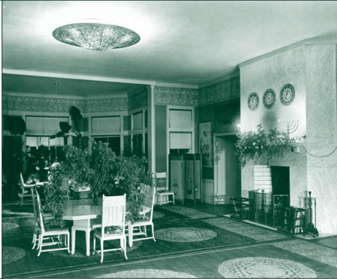
Dining room, Laurelton Hall, c. 1925. Photograph by David Aronow.
