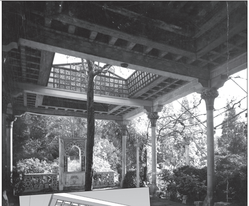
Above: View of the Daffodil Terrace showing ceiling, column capitals, and the iridescent-glass skylight through which a pear tree grows.
