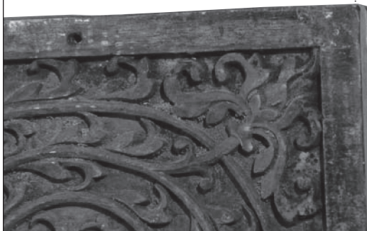
Left: Ceiling tile detail from the Daffodil Terrace. The molded floral tiles were cast of a composite material from carved hardwood originals. Above top: Another coffer tile design. Trying to visualize the ceiling as Tiffany might have, conservators arranged and rearranged its parts until patterns emerged. Above: One of hundreds of iridescent-glass tiles from the terrace's pear-tree skylight.
