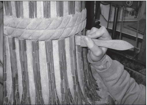
The daffodil stems are formed of glass tesserae. During cleaning, conservators discovered watercolor washes on the mortar between the stems nearest the flowers.
