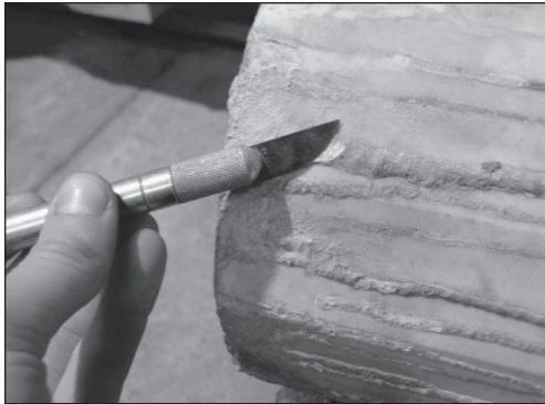
Removing mineral buildup from the terrace's column shafts was an extremely time-consuming process.
