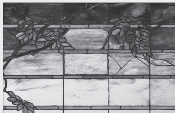
Above: Magnolia window, c. 1885. Conservation: Replace frame, clean, correct bowing, replace previous repairs with original Tiffany glass.
