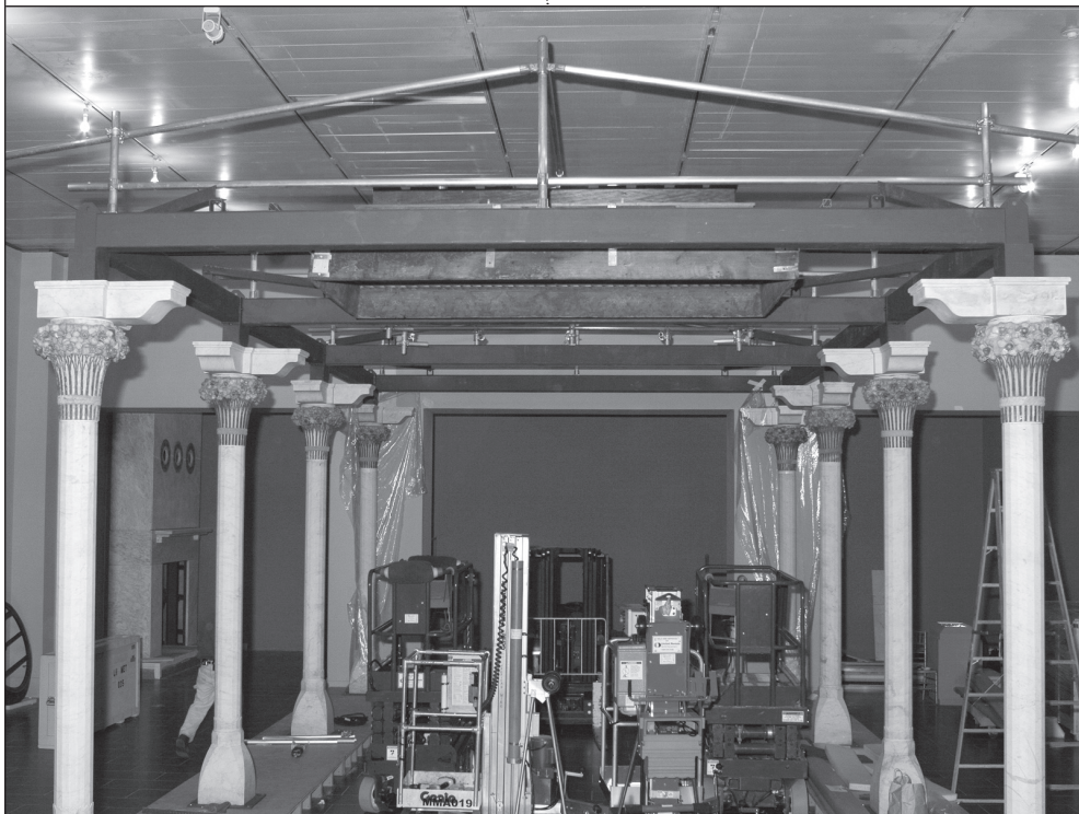
The installation of the components of the Daffodil Terrace began at the Metropolitan in mid-October. The marble mantelpiece from the Laurelton Hall dining room can be seen in the background. Photo by Wallace Lewis, Metropolitan Museum of Art.
